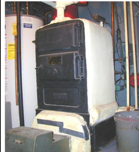
A typical boiler covered with Asbestos Cement
