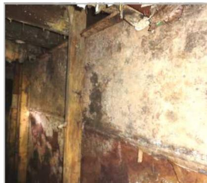
Mold growing on a basement/crawlspace wall.
