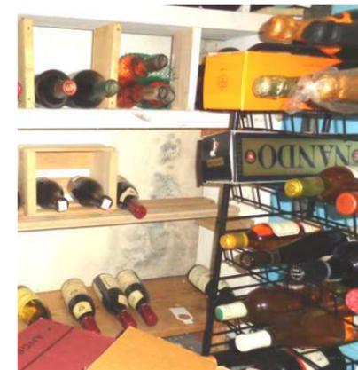
Mold and Water Damage behind shelving.
