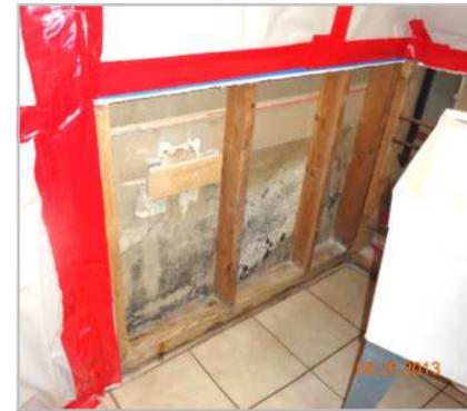
Mold growth inside wall cavity. Room is prepared for remediation.
