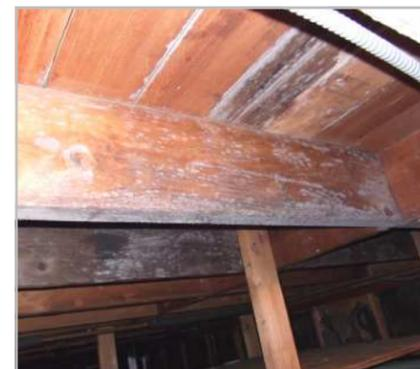
Mold impacted floor joists and sheathing.
