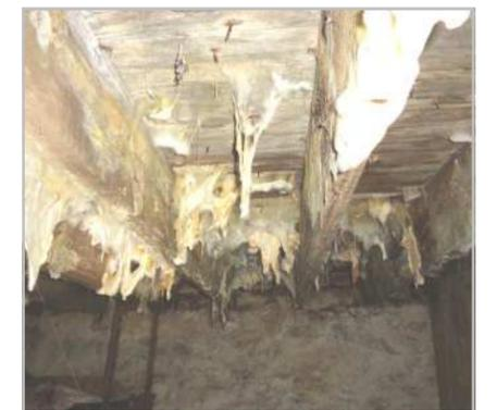
Mold Impacting Basement Ceiling Joist. Possible water leak from Bathroom above.
